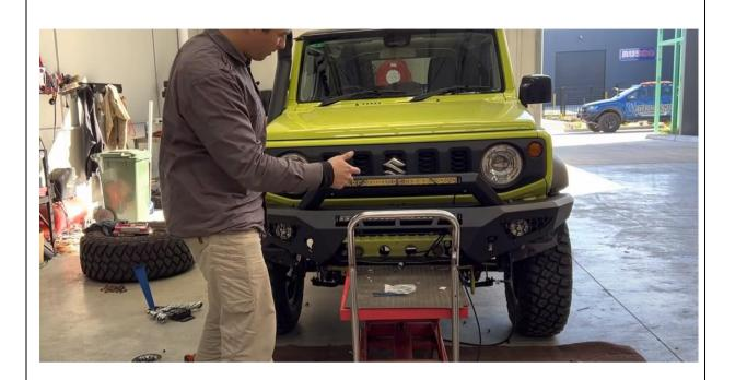
47. Using a lifting trolley, trolley jack or mate lift bar onto the mounts and secure with M10 x 30 bolts, flat washers and Nyloc nuts
