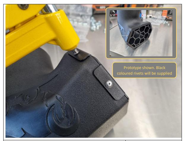
106. Fit the B-1260 air ram mesh piece to the air ram body and insert 4x black size 4-4 pop rivets.
