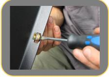
85. Fit 5x Cage nuts from small parts kit to rectangular slots in bottom of wing.
