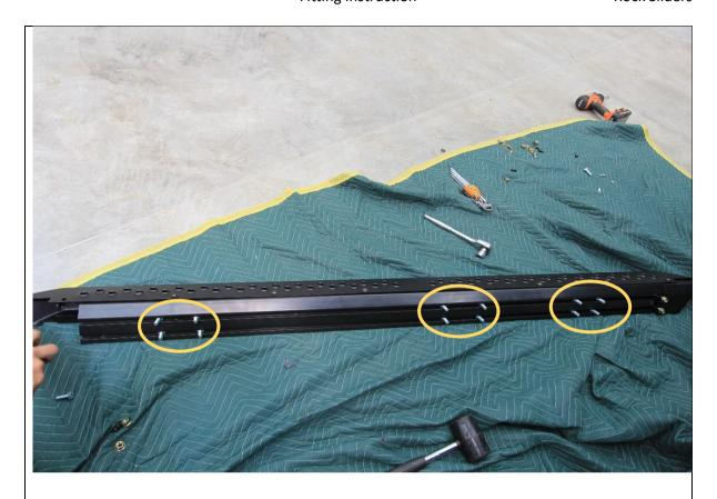
35. Slide the 12x M10x25 Hex bolts into the T slots on back side of extrusion. 6 bolts per slot.
